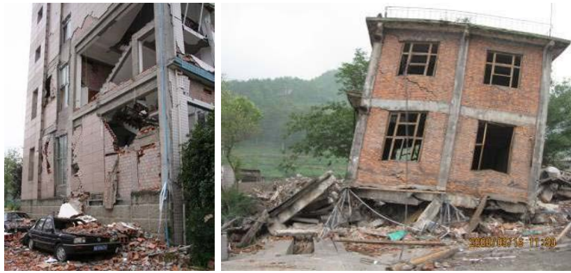
Figure 1. Infill masonry walls performance at Wenchuan Earthquake [3].
