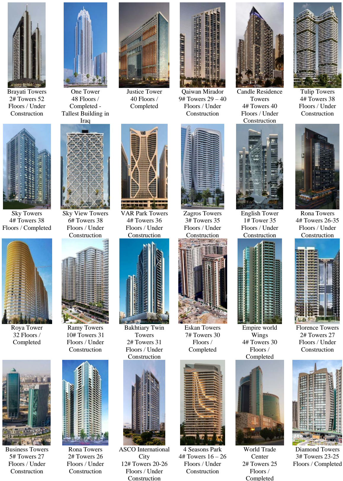
Figure 1. Some of the Erbil Towers constructed or under construction.
