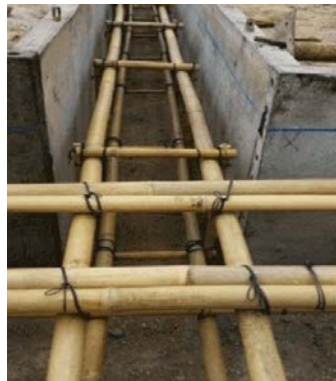
Figure 2. A practical example of developing countries using bamboo-reinforced concrete
